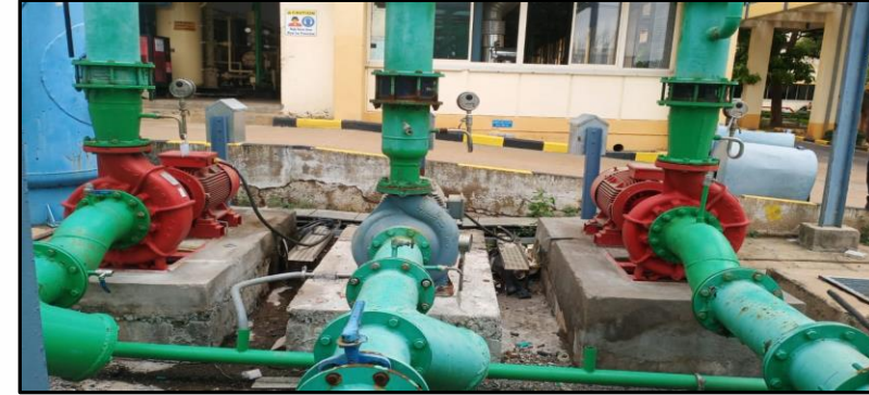
REPLACED CONDENSOR PUMPS WITH ENERGY EFFICIENT MOTORS.
